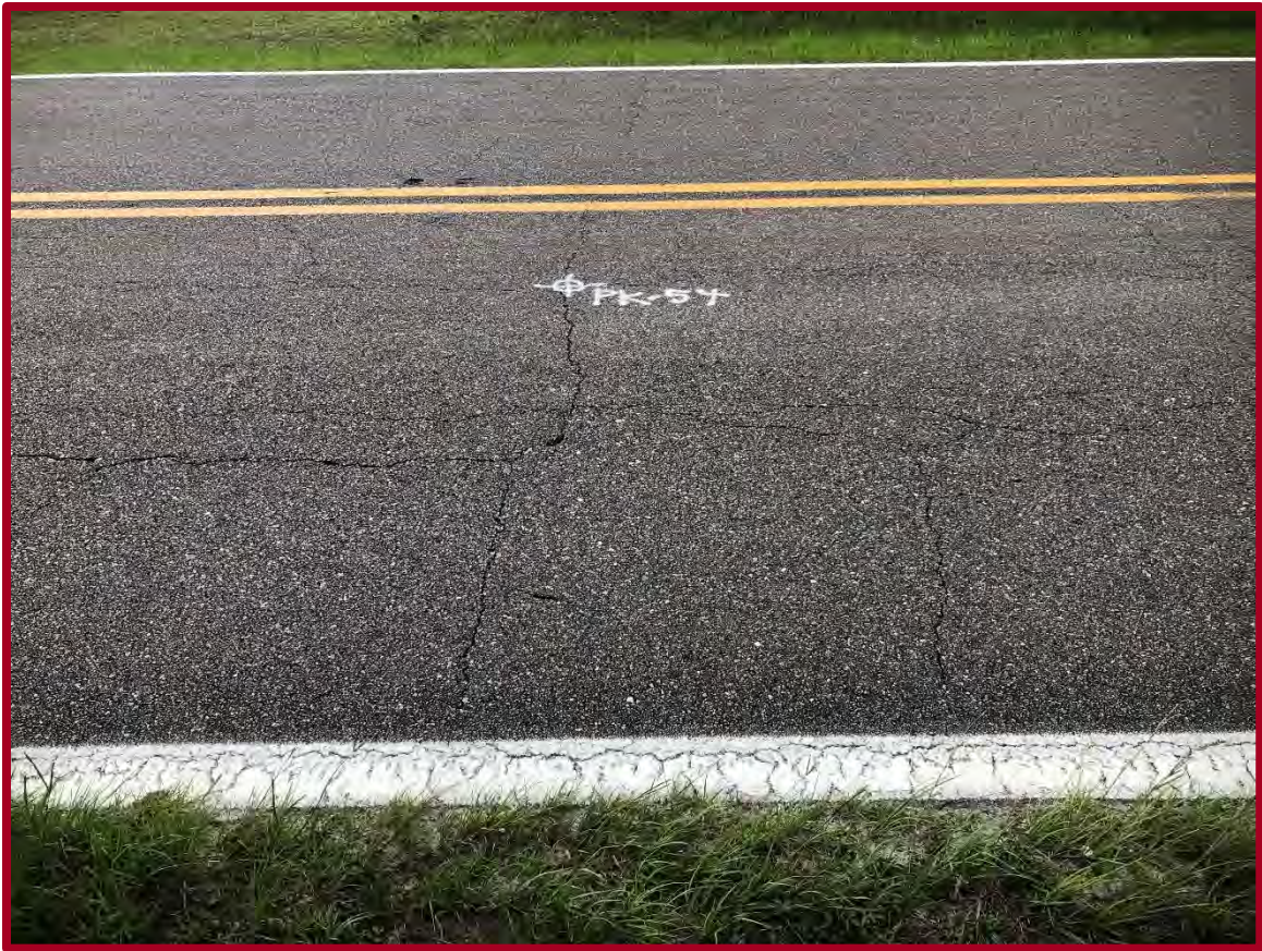
FIGURE D107: EXISTING CONDITIONS AT PAVEMENT CORE PK-54 (FACING SOUTHWEST)
